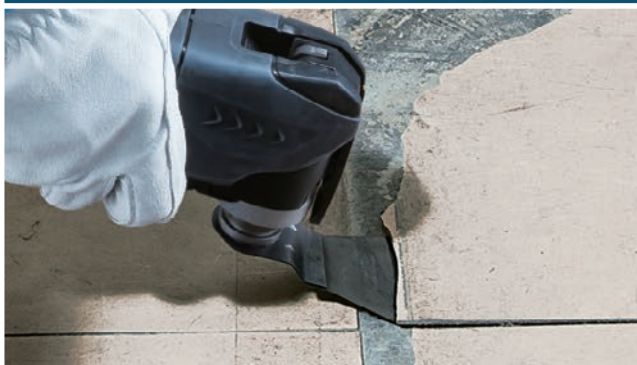
Scraping floor tiles
