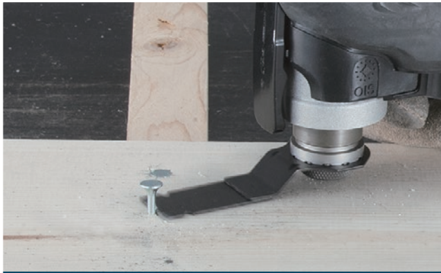
Flush cutting of nails
